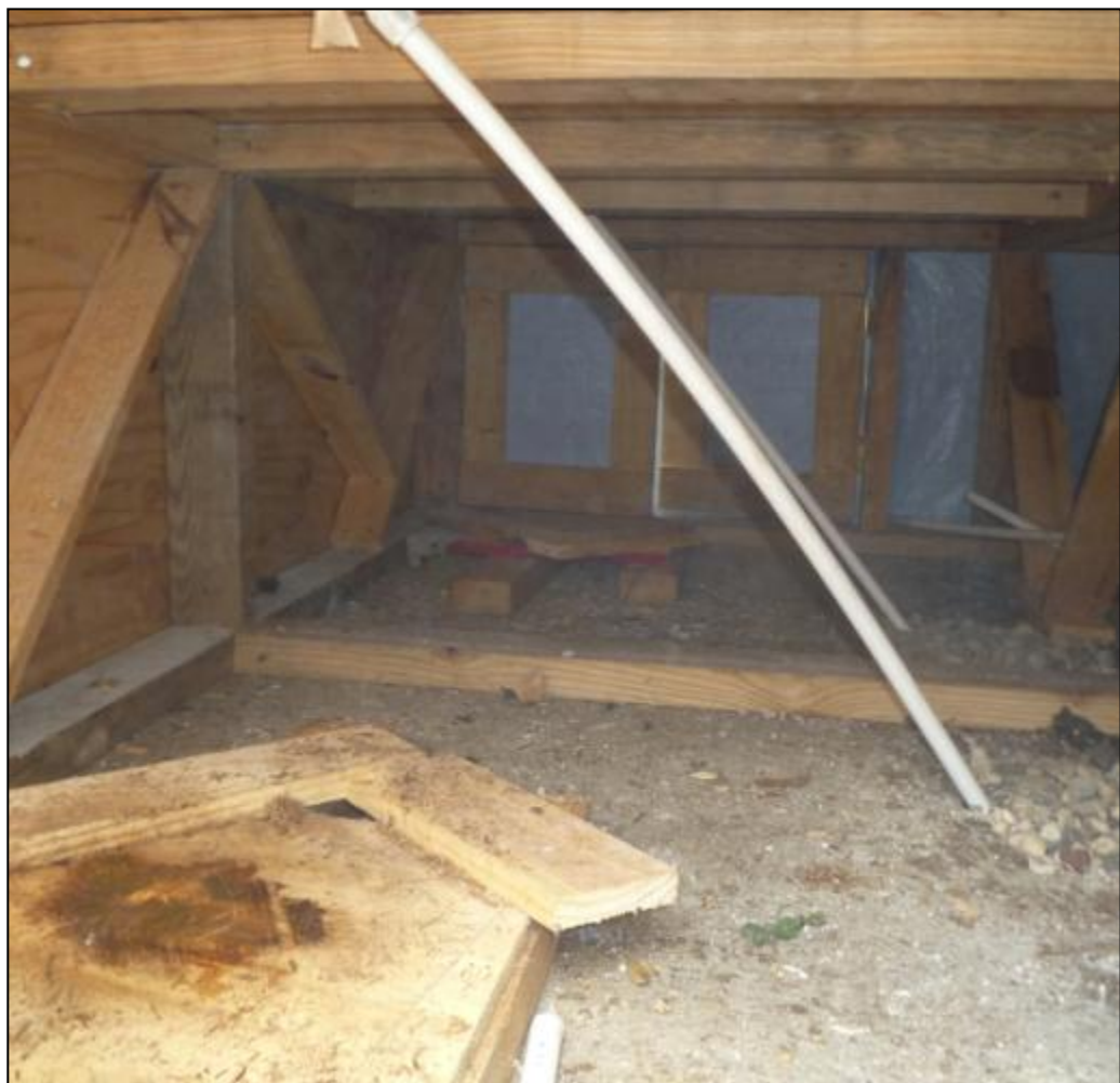
PHOTO T1: Chamber beneath toilet
