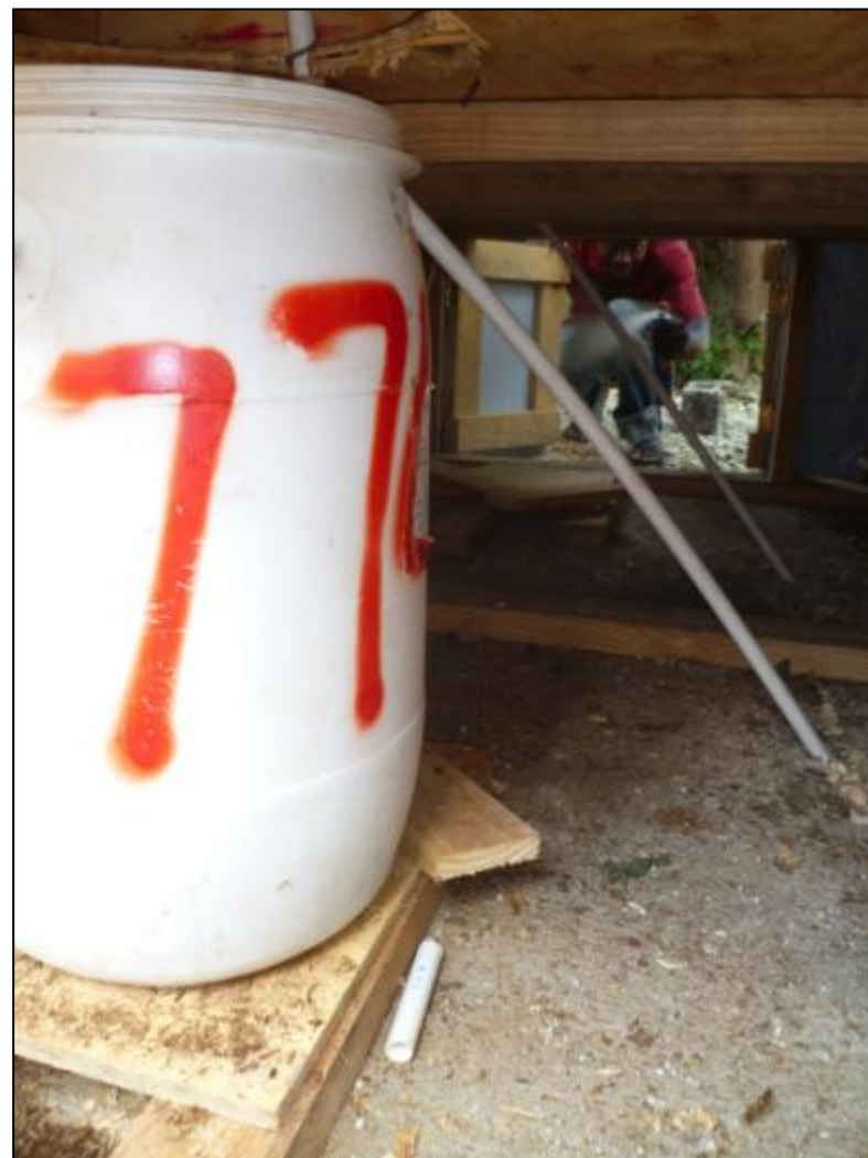
PHOTO T2: Drum in position beneath poophole
