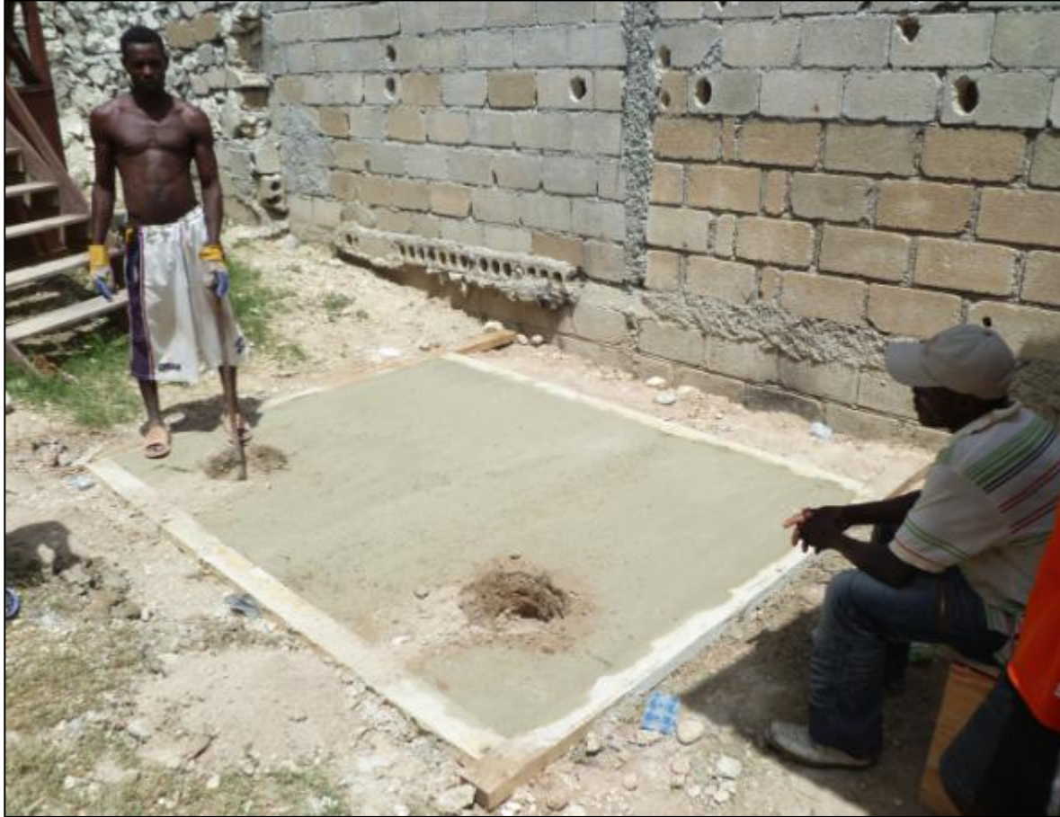
PHOTO T3: Digging urine soakaway pit after concrete base construction
