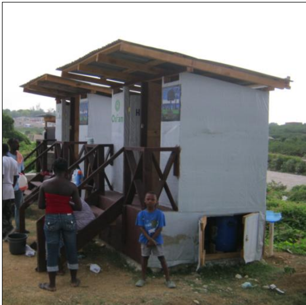
PHOTO T11: Sideview of toilet showing chamber doors
