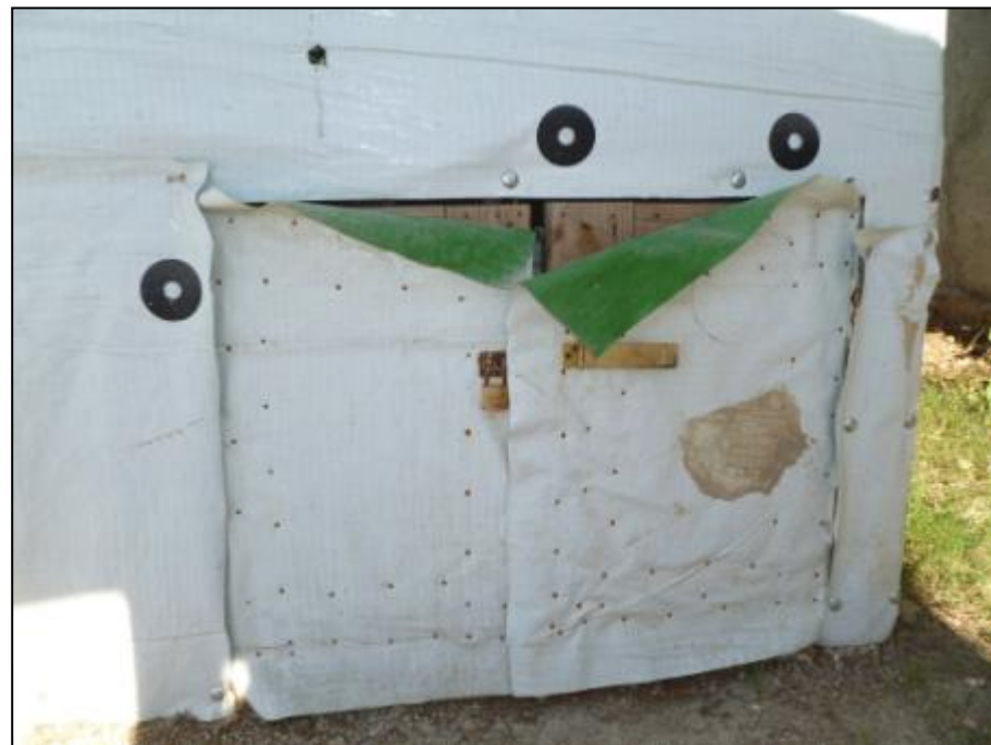
PHOTO T12: Close-up on chamber doors
