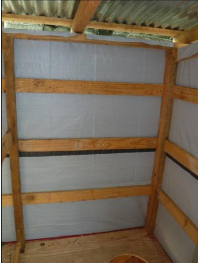
PHOTO T9: Internal Walls
