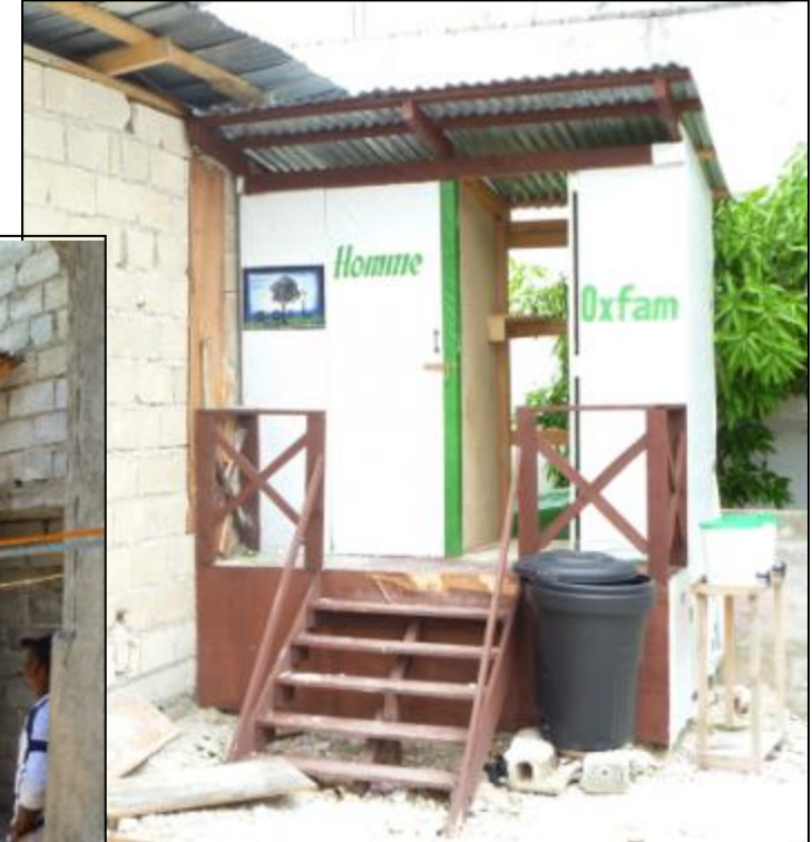
PHOTO T16c: BAD positioning of SOIL UD toilet with not enough space for chamber access
