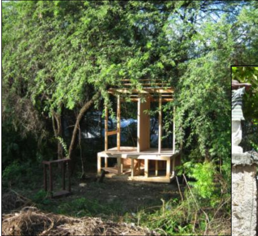
PHOTO T16a: SOIL UD toilet positioned in shade. Positioned for privacy, but too obscure?
