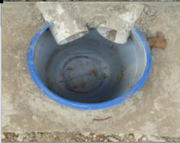
Photo K108: Leachate drain from 2 compost compartments collected in a single 15 gallon drum
