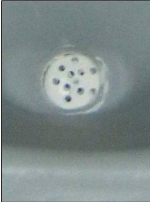
PHOTO BAD T4a: Early SOIL UD toilet seat with holes for urine drainage, NO filter.
