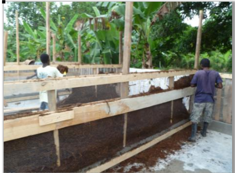
Photo K113: Filling bagas walls BEFORE drum dumping begins
