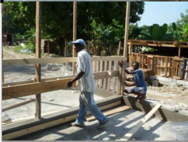
Photo K112: Interior walls construction.
