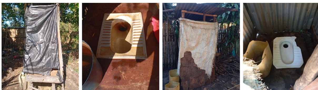
Figure 14. Overview of improved toilet stalls made of light materials (Source: Practica)
