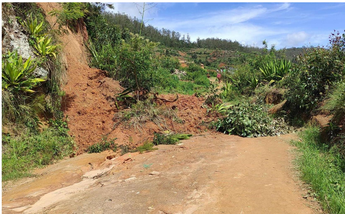
Figure 13. Landslide cutting access to the STBV after heavy rainfall in 2021 (Source: Practica)
