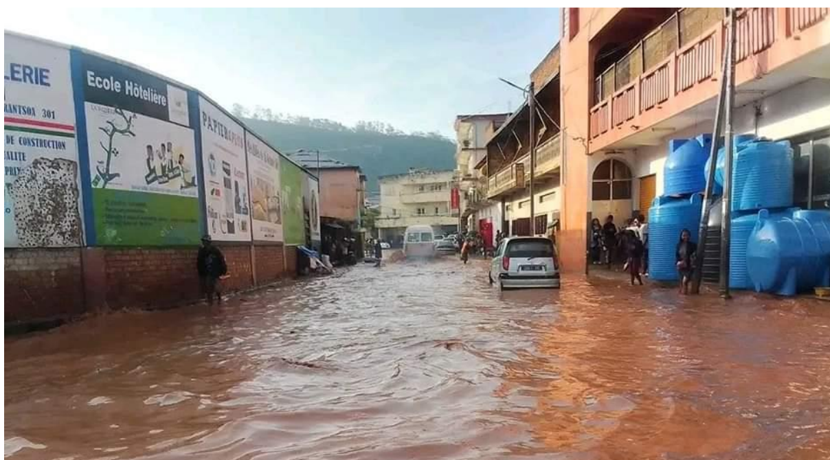
Figure 7. Overview of Flooding in Fianarantsoa Following Cyclone Batsirai in 2022 (Source: BNGRC)
