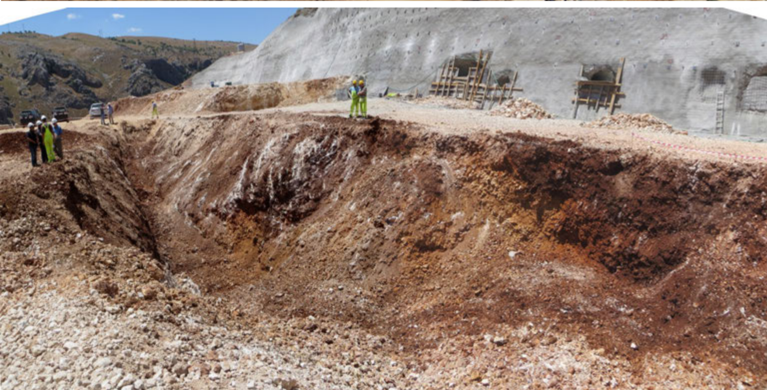
Slope protection & excavation for foundation of Headworks structure
