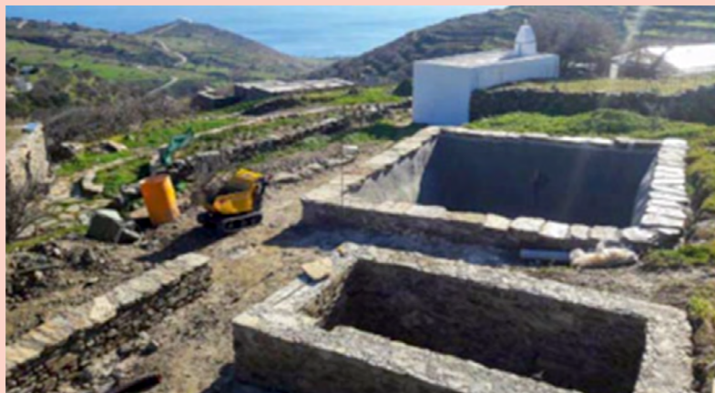
Constructed wetland and rainwater tanks under construction
